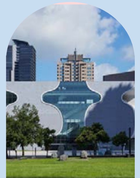
Photo from National Taichung Theater
